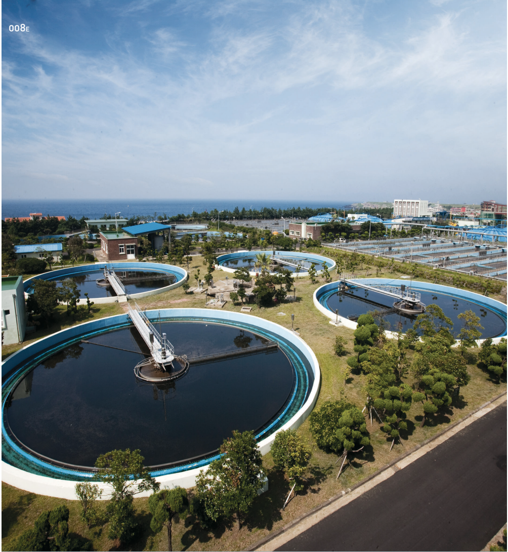
008e Jeju Advanced Sewage treatment plant
