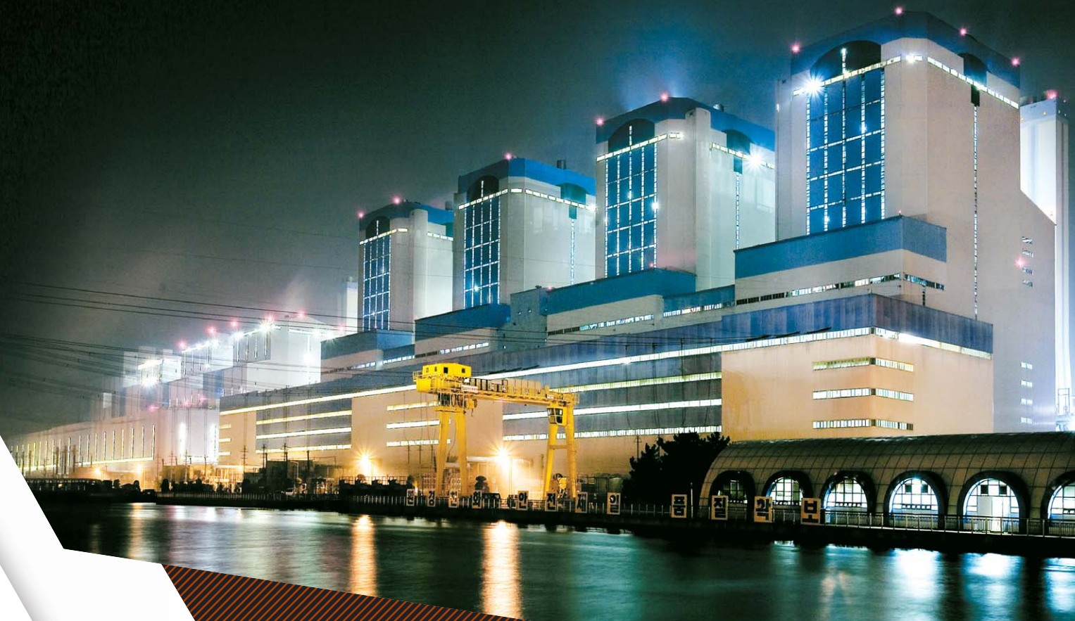
Dangjin Coal-Fired Power Plant(Unit 7 & 8)
