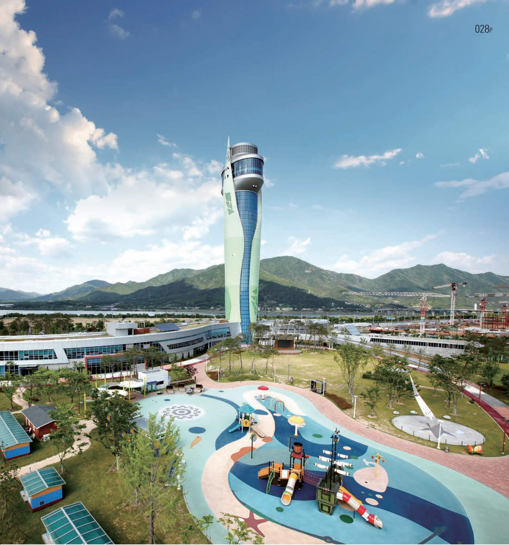
026P Jecheon Municipal Solid Waste Treatment Plant Location: Jecheon, Korea - Incineration plant: 50 ton/day - Stoker type Project period: 2006. 03 ~ 2008. 08
