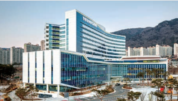
Changwon Gyeongsang National University Hospital (BIM+LEAN)
