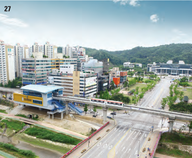
27. Uijeongbu Light Railway Transit Location: Uijeongbu, Korea - Total Length 11.1km - 15 Stations, 1 Depot Project period: 2007.08 ~ 2011.07 28. Electrified Double Track Railway in Jungang Line (Cheongnyangri-Deokso Sec.) Location: Namyangju, Korea - Total Length 9.5km, 15 Bridges (1.97km) - 4 Stations Project period: 1997.10 ~ 2006.06
