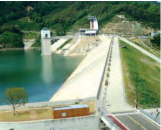
Renewable (Pumped Storage Hydroelectricity)
